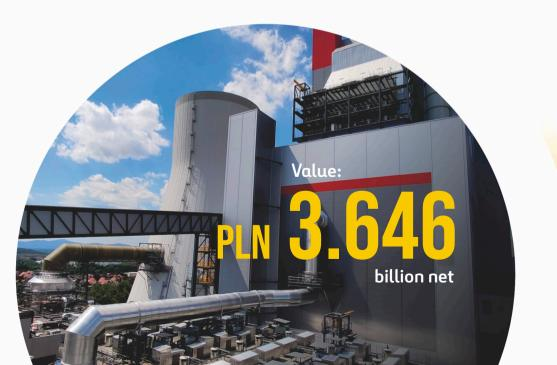
As part of a consortium with Mitsubishi Hitachi Power Systems Europe GmbH and Tecnicas Reunidas S.A., we built a separate 450 MW power unit, which operates on supercritical steam parameters. The generating unit is a single-pass tower flow boiler with a pulverised fuel furnace and a low-emission combustion chamber, in combination with a condensing steam turbine.
